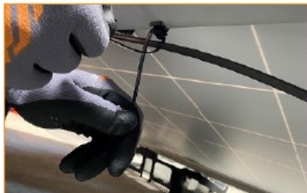
Examples of wire installation under module frame.
