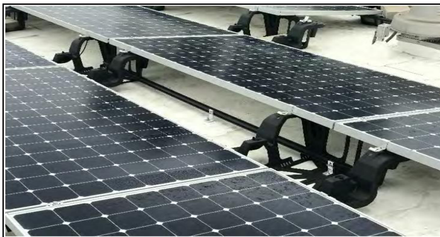
Figure 4- Mechanical Anchor Assembly
