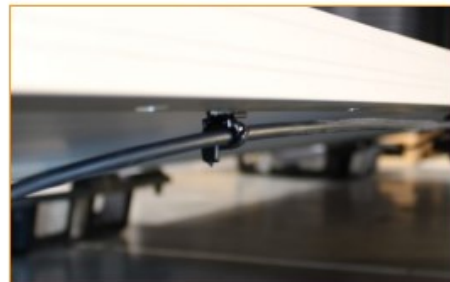
Examples of wire installation under module frame.
