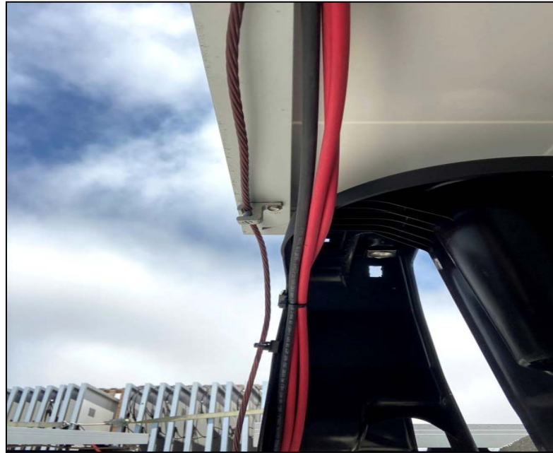
Figure 8-Nylon Wire Management Zip-tie Clips (FR-W-CLP)
