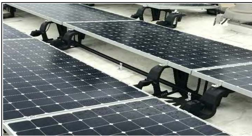
Figure 4- Mechanical Anchor Assembly
