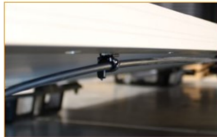
Examples of wire installation under module frame.
