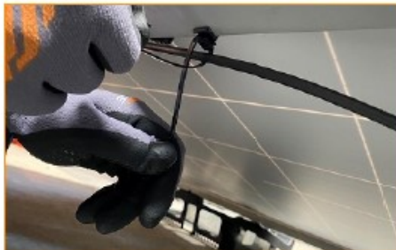
Examples of wire installation under module frame.
