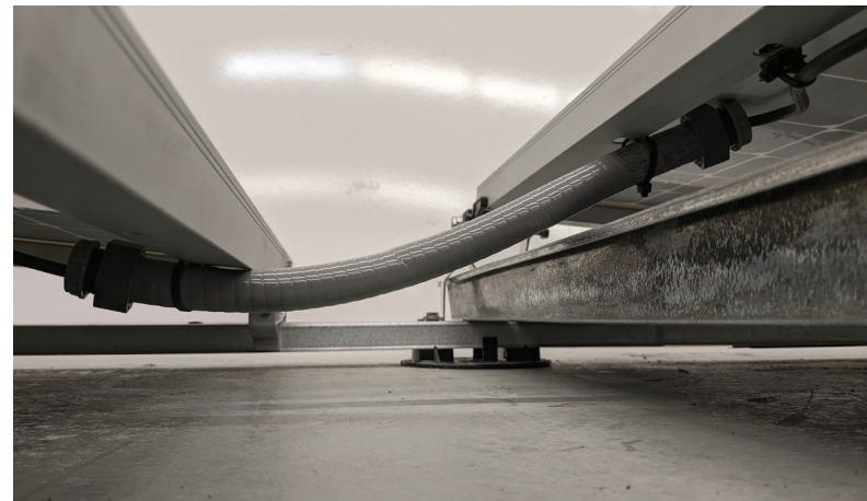
OPTION 2: USING FLEXIBLE NONMETALLIC CONDUITS
