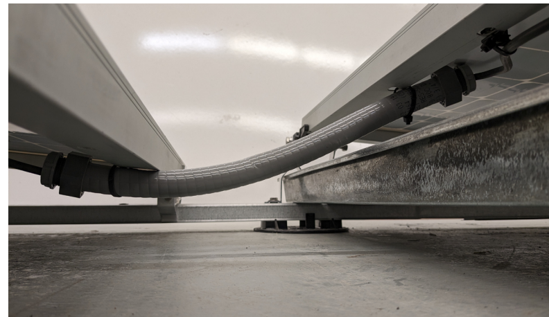
OPTION 2: USING FLEXIBLE NONMETALLIC CONDUITS
