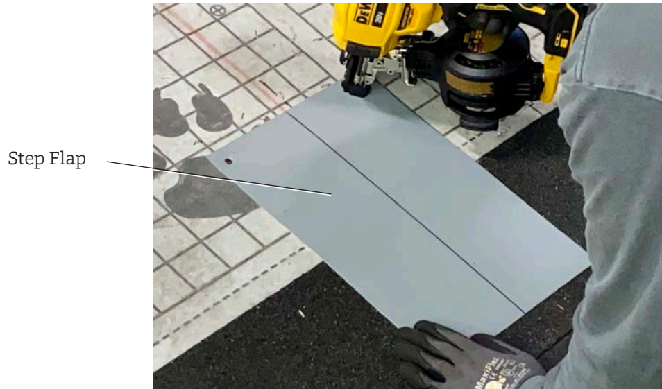
Figure 10. Nail Step Flap in place
