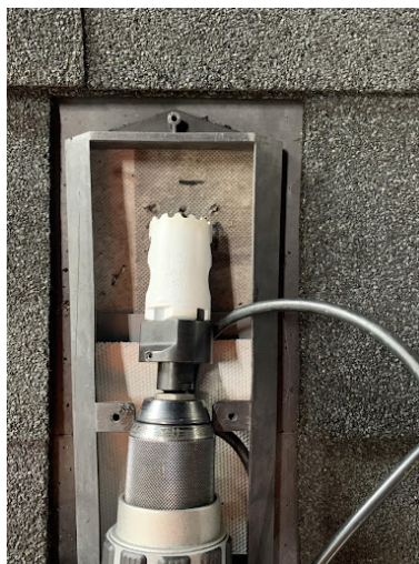
Figure 34. Installing Pass Through Device
