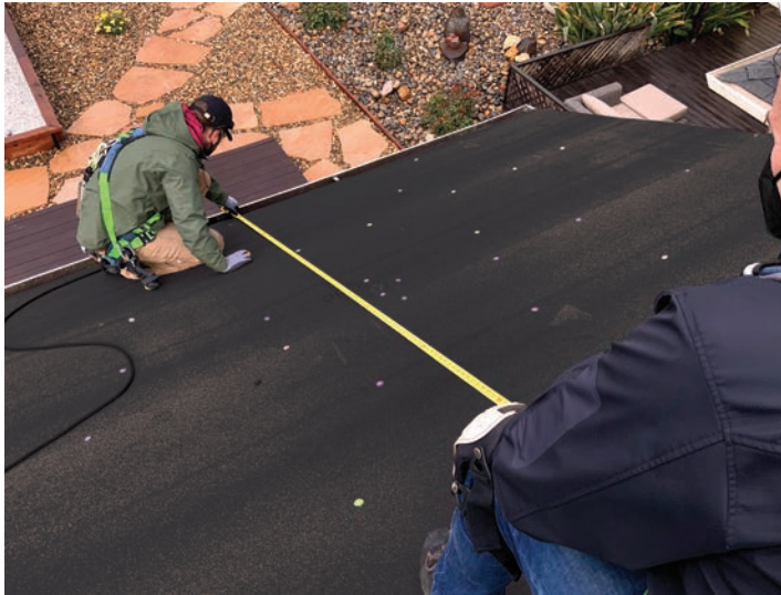
Figure 4. Compute array dimensions
