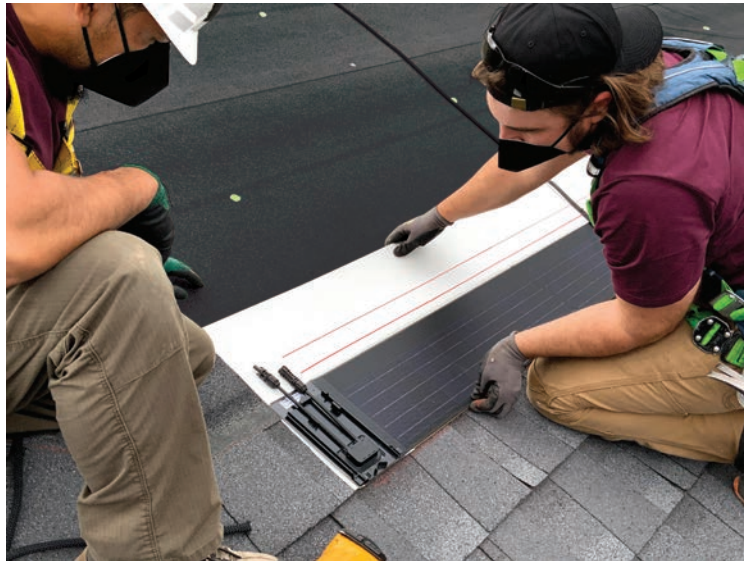
Figure 11. Install first Solar Shingle
