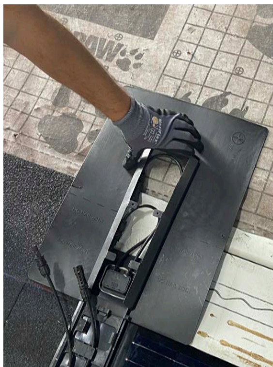
Figure 21. Align Top Flashing
