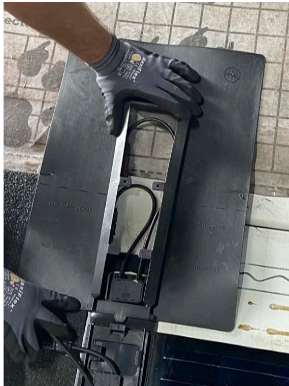
Figure 20. Position Top Flashing
