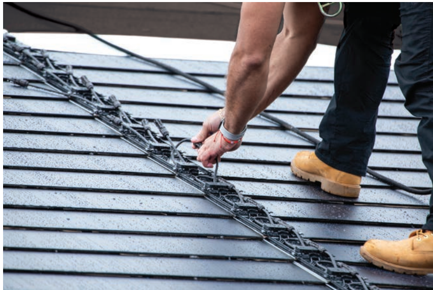
Figure 17. Ensure that vertical wire channels are straight
