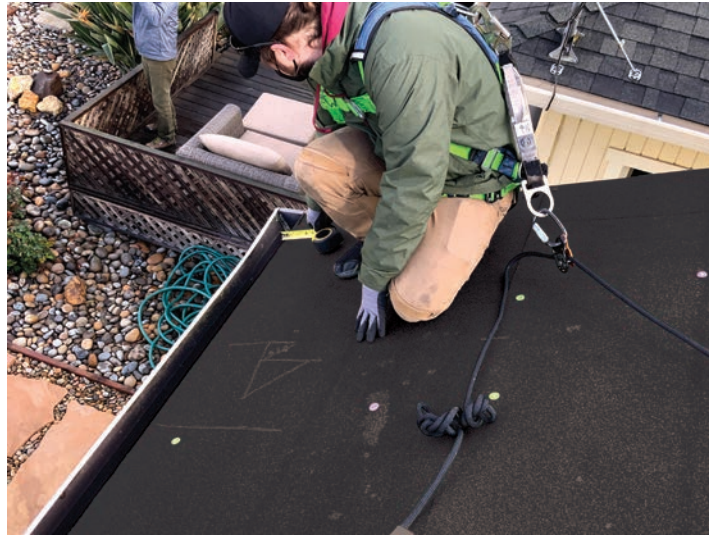
Figure 6. Locate array starting point
