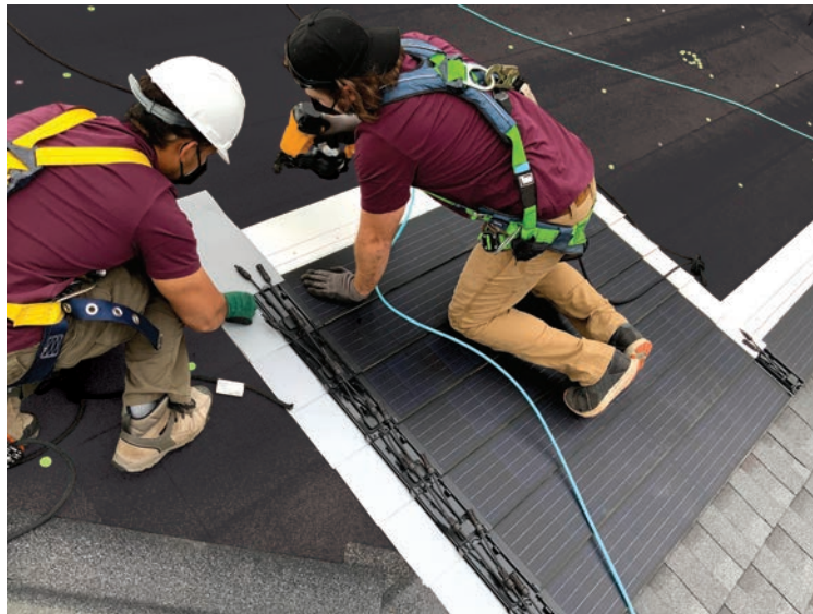
Figure 14. Step Flaps going up the column
