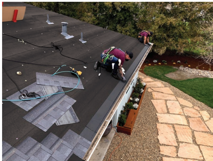
Figure 7. Bottom course of roofing shingles
