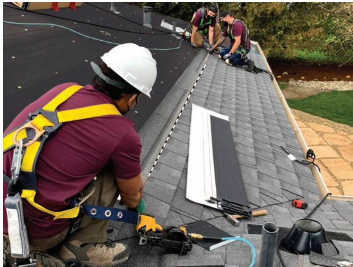
Figure 8. Snap horizontal chalk line along array bottom edge
