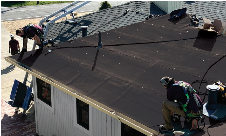
Figure 3. Install roofing underlayment
