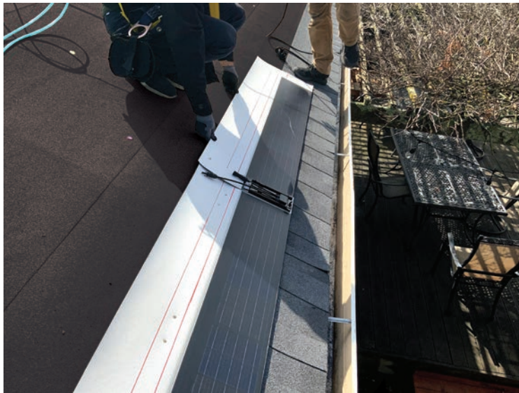
Figure 12. Install next Solar Shingle
