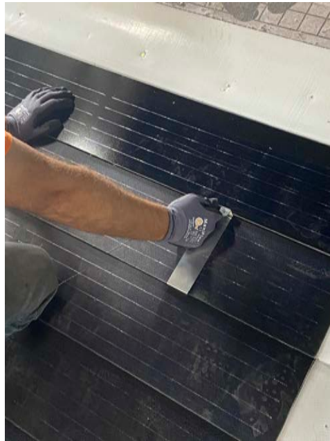
Figure 15. Next Solar Shingle going up the column
