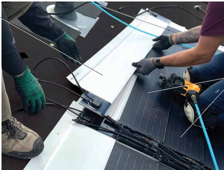
Figure 18. Position a Jumper Module at top of columns, per plan set
