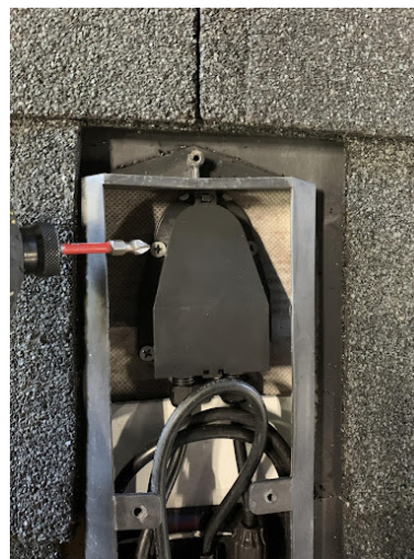
Figure 34. Installing Pass Through Device
