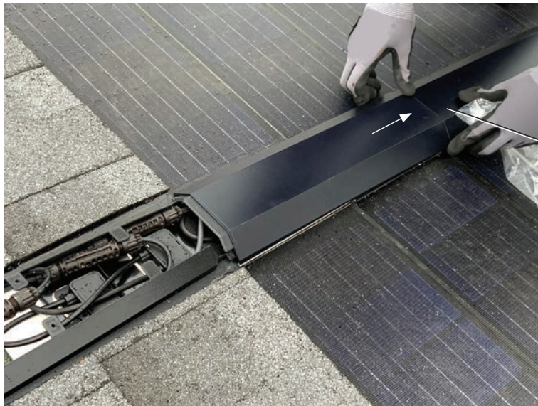
Figure 25. Use built-in wire clip features to secure wires
