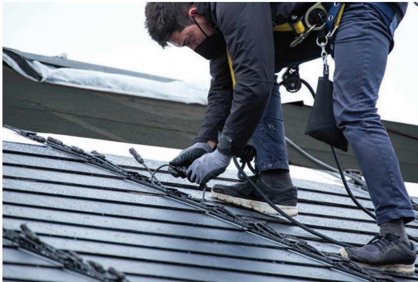
Figure 23. Connect Solar Shingles
