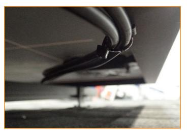
When running wires north/south or east/west under a module, attach Edge Clip or other approved positioning device to module frame flange and use Cable Tie to secure wires to module frame, where needed. Cut off any remaining cable tie after installation, where needed. All wires must remain underneath the module after installation.
