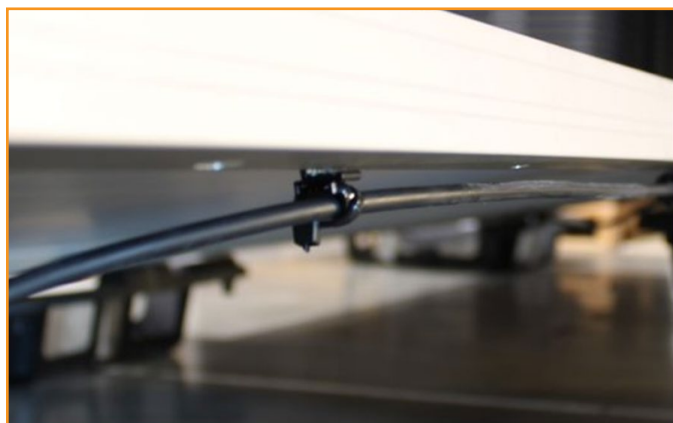
Examples of wire installation under module frame.
