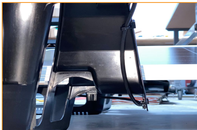
Examples of wire installation under BX Chassis.
