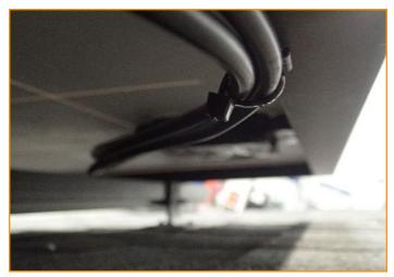
When running wires north/south or east/west under a module, attach Edge Clip to module frame flange and use Cable Tie to secure wires to module frame. Where needed, cut off any remaining cable tie after installation. All wires must remain underneath the module after installation. There shall be no visibly exposed wires after installation of modules.
