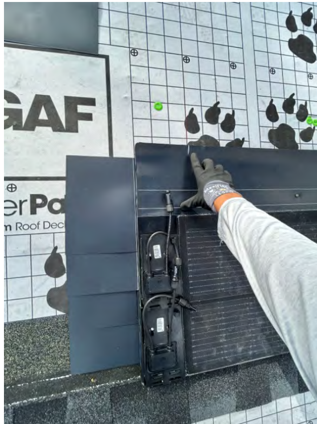
Figure 26. Next Energy Shingle going up the column
