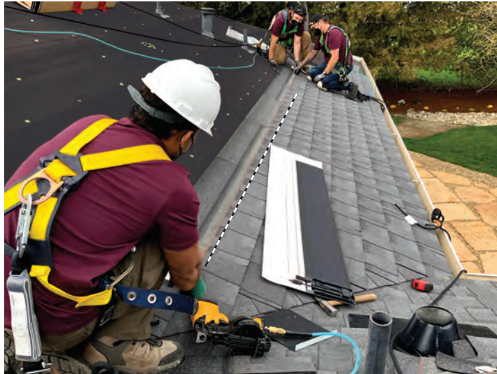
Figure 20. Snap horizontal chalk line along array bottom edge
