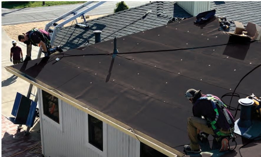
Figure 15. Install roofing underlayment
