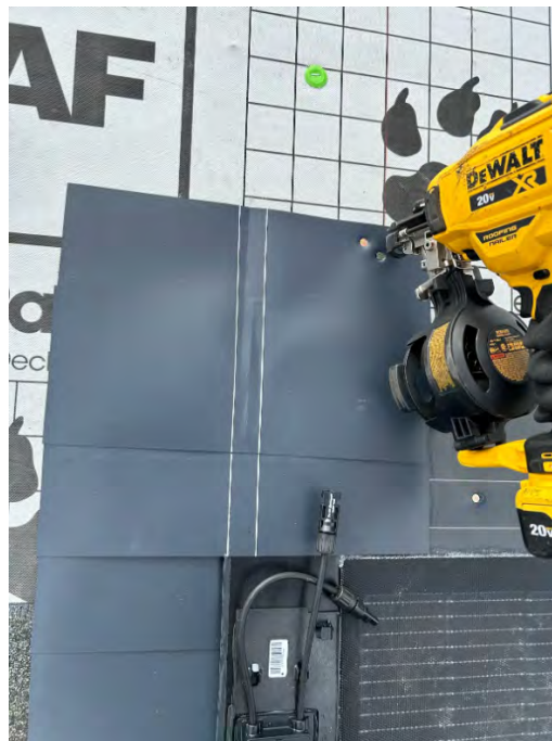
Figure 30. Continue step flaps for the JM on the left edge of the array
