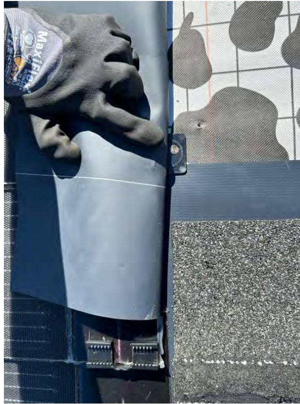
Figure 37. Install and nail floating bracket underneath right side flap and step flap
