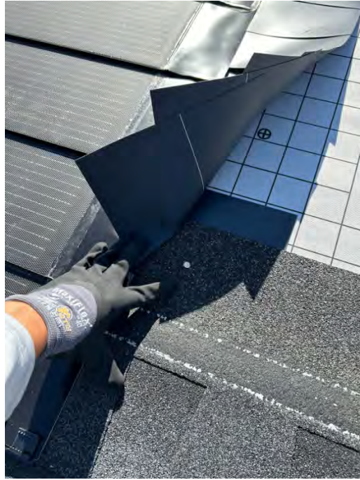
Figure 39. Lift the step flap when nailing the asphalt shingle
