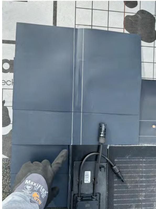
Figure 25. Align the next step flap up the column
