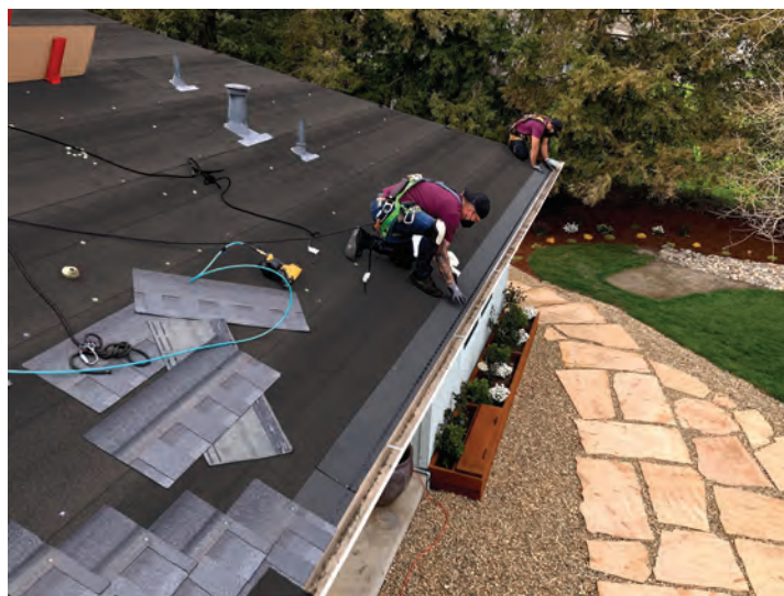
Figure 19. Bottom course of asphalt shingles
