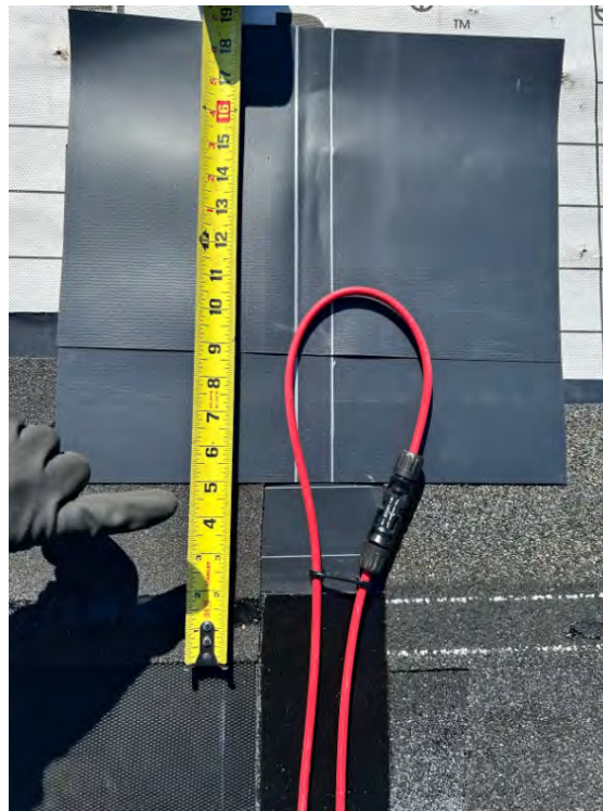
Figure 42. Install step flaps at the top of every wire channel
