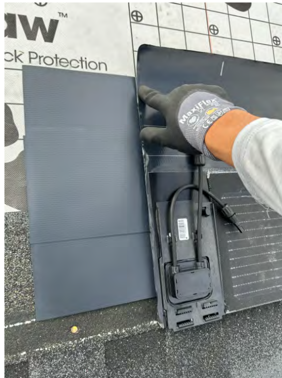
Figure 24. Install the first Energy Shingle
