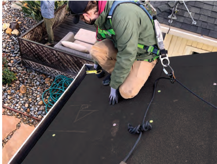
Figure 18. Locate array starting point
