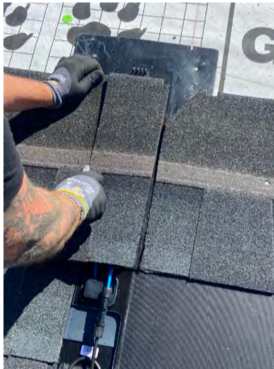
Figure 45. Cutting shingles around top flashing
