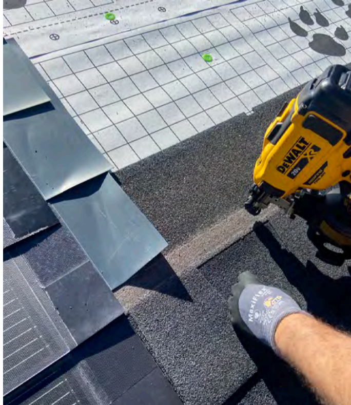
Figure 38. Butt asphalt shingle to the right side flap
