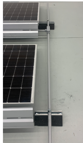
OPTION 2: USING RIGID NONMETALLIC CONDUITS
